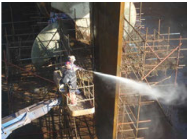
Washing the vessel before painting
